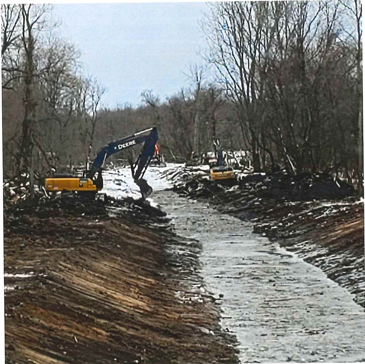
Tebo-Erickson Drain Project
